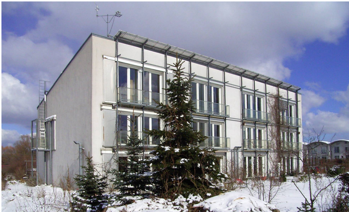
Figure 2: The first Passive House in Darmstadt-Kranichstein which was used as an example in this study
